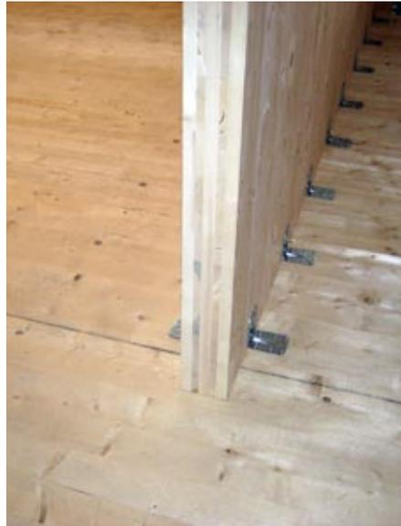
Wall panel anchored to floor panel.
